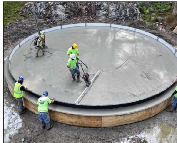
Reinforced concrete floor with embedded starter ring
