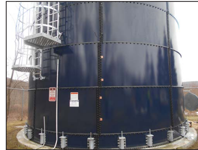
Expanded tank with two new rings at bottom
