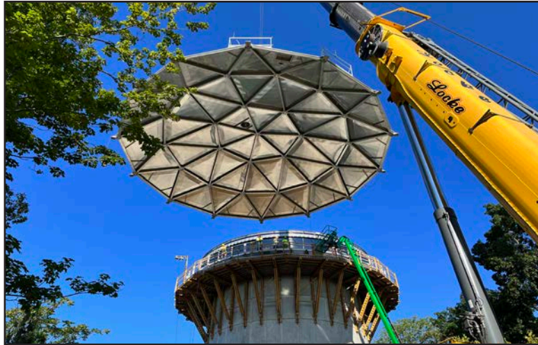
Crane placement of a CET geodesic dome
