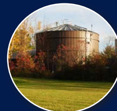
Aerobic & Anaerobic Digesters
