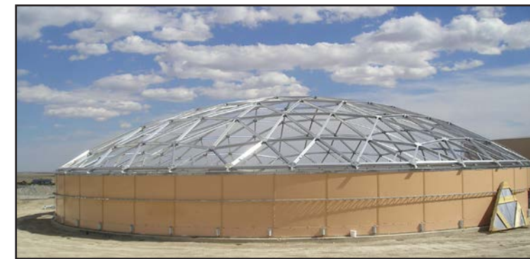
Geodesic dome prior to aluminum panel installation
