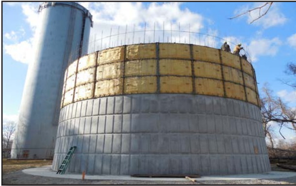
CET construction with jump forms
