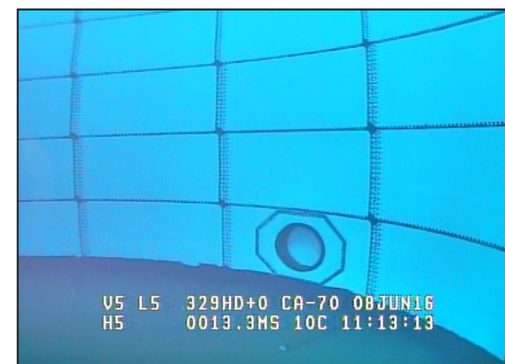
AQUASTORE® tanks have a white interior making them easy to inspect
