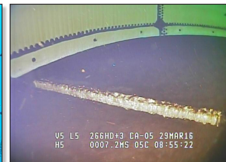
Submersible inspection of cathodic anode
