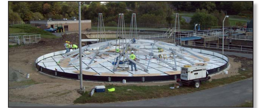
Geodesic dome construction at ground level
