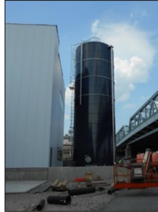
Tight footprint installation
