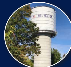
Composite Elevated Tanks (CET)
