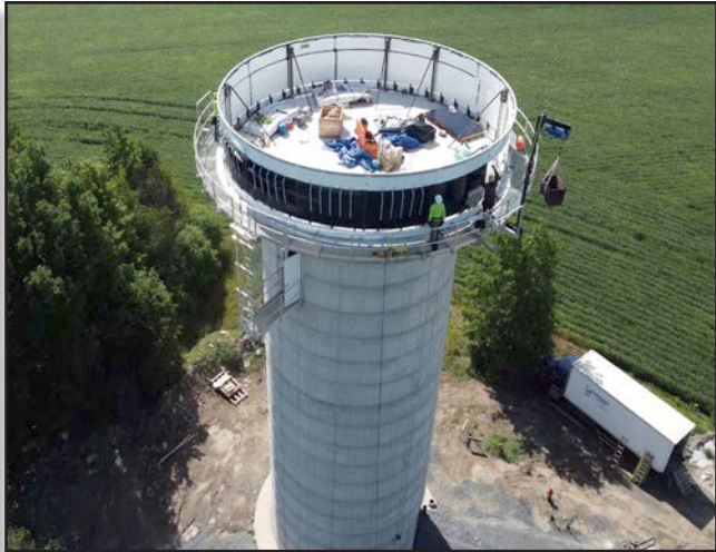
CET with pan and initial tank construction
